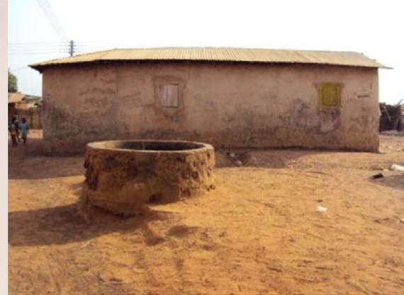
Image 6: borehole in Wulensi, Northern Ghana, built by an NGO, but no longer functioning
